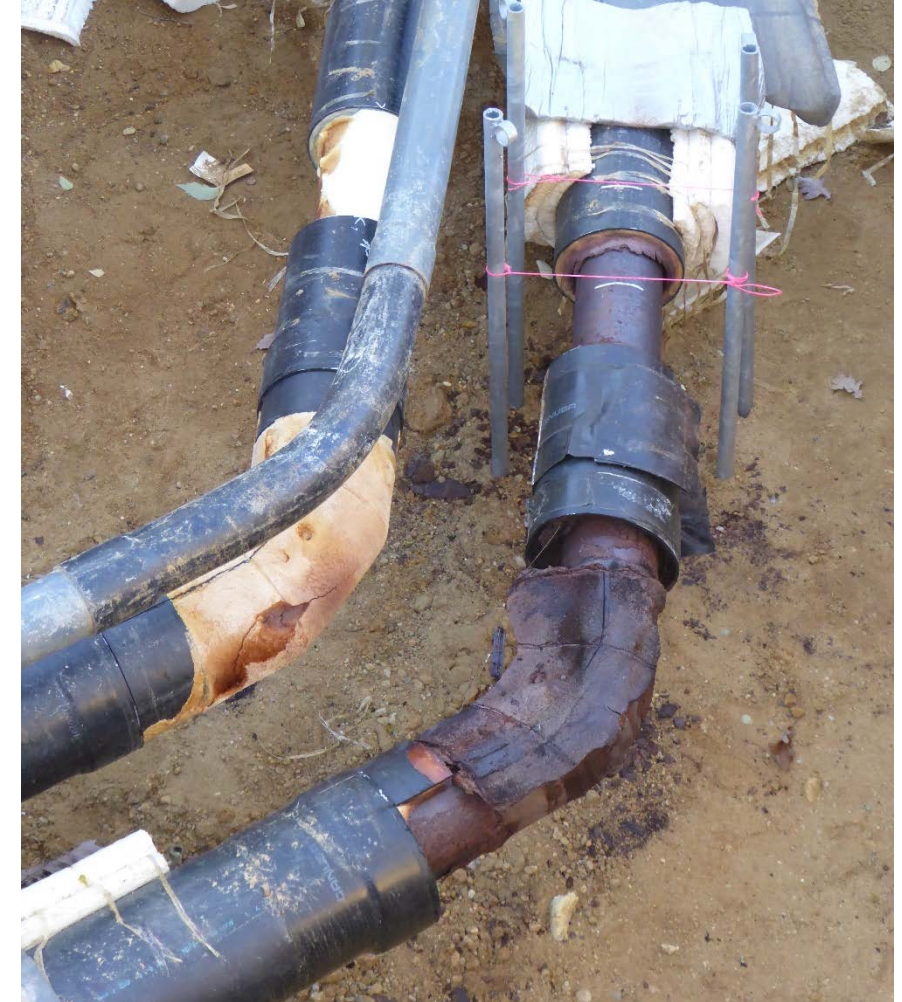
Measurements on a heating network with insufficient connection of the DH pipes, Source: AGFW
