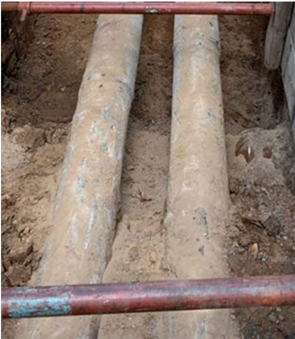
Removal of test specimens FWA - straight pipe and 90° bend, Source: AGFW Documentation sheet for the FWA sampling point, Source: AGFW
