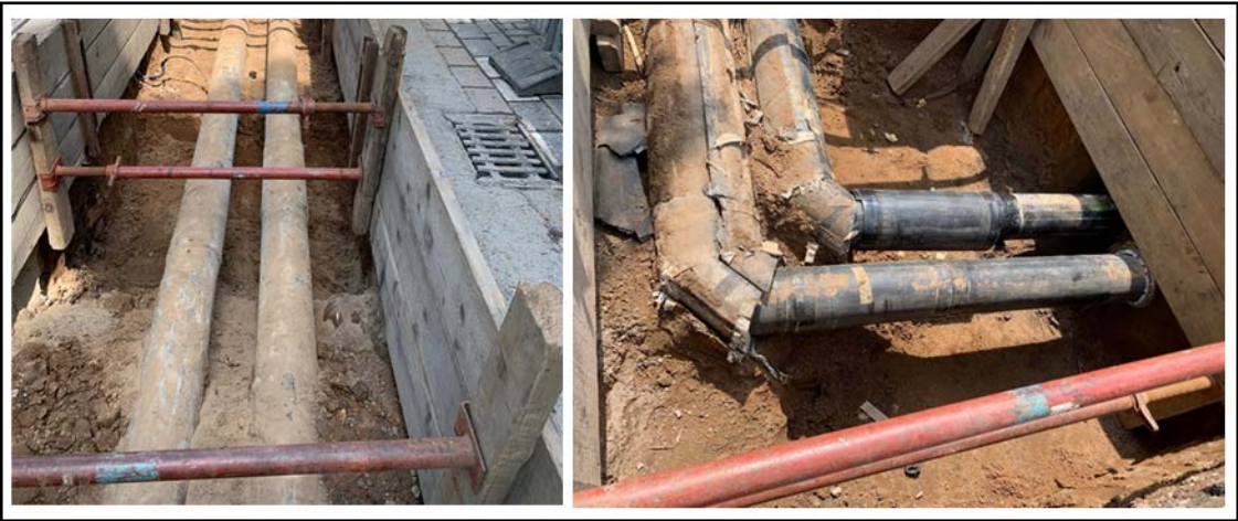
Removal of test specimens FWA - straight pipe and 90° bend, Source: AGFW
