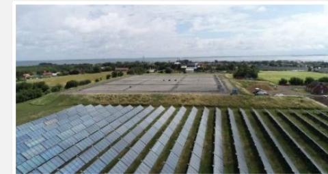
Overview of solar heating systems and Pit Thermal Energy Storage at Marstal district heating plant.
