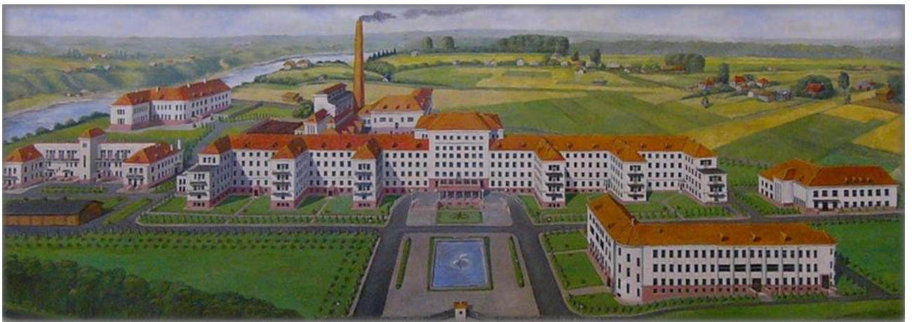
Fig. 1 The building complex of the Vytautas Magnus University Medical Campus (Clinics) in Kaunas
