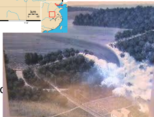
Shimantan Reservoir Dam
