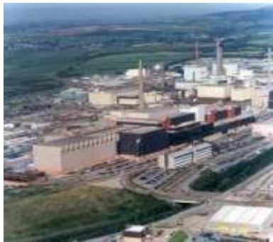
Spent fuel reprocessing - THORP, MAGNOX & associated plant
