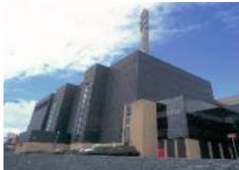
Waste and effluent treatment plants
