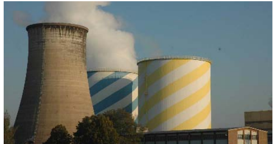
Combined heat and power plant "Chemnitz North II"
