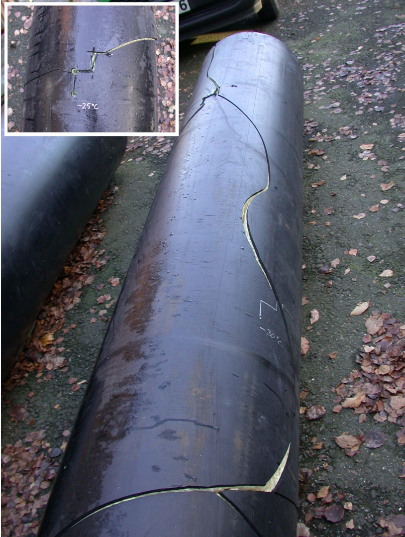
Figure 5. After handling test at -25 °C with fracture on material B.
