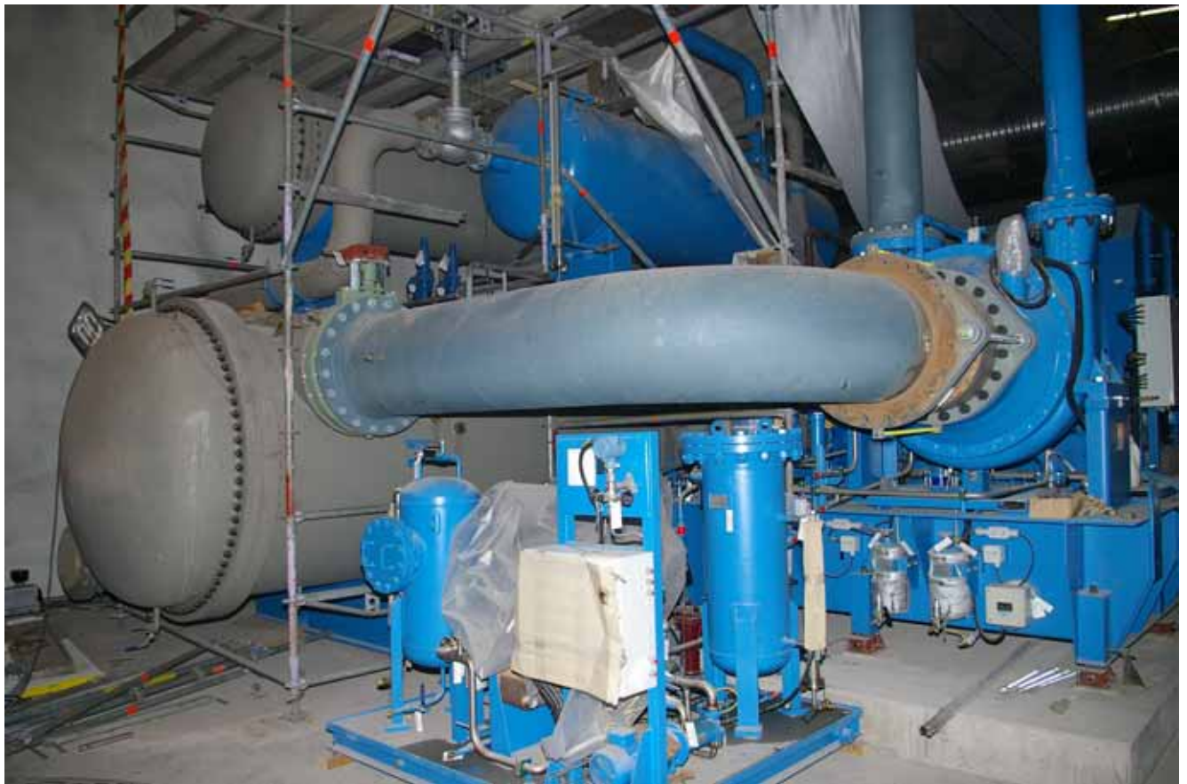
Heat pump UNITOP 50FY during assembly on site
