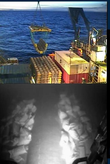
Concrete mattresses under and on the cable at a depth of 60 m
